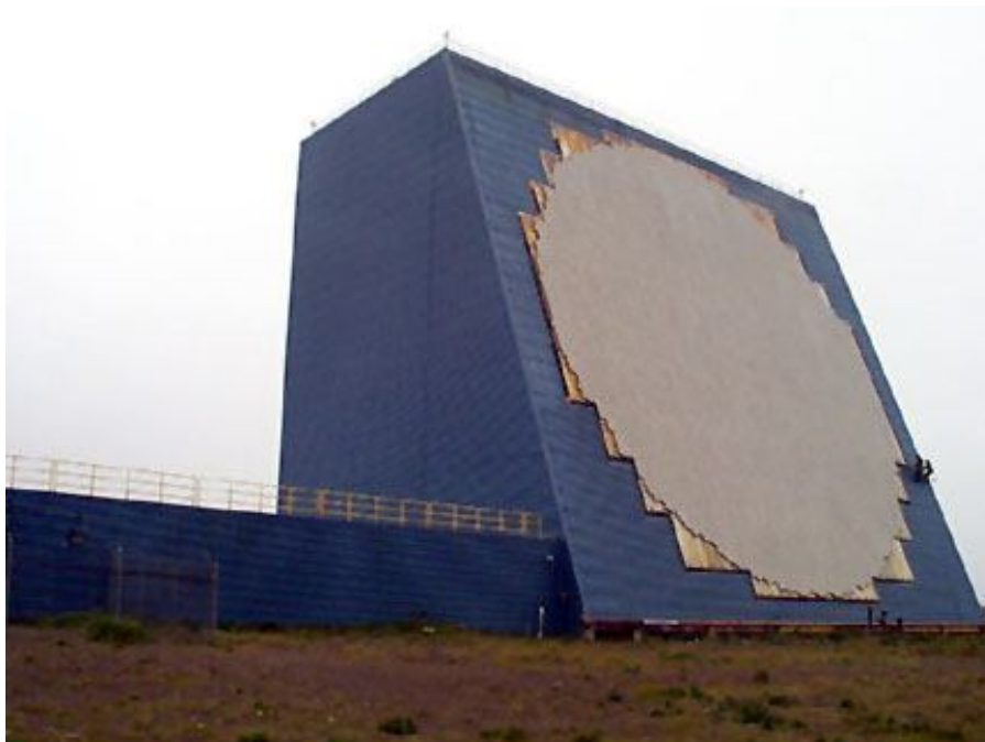
Picture 20. Cobra Dane-radar 27
