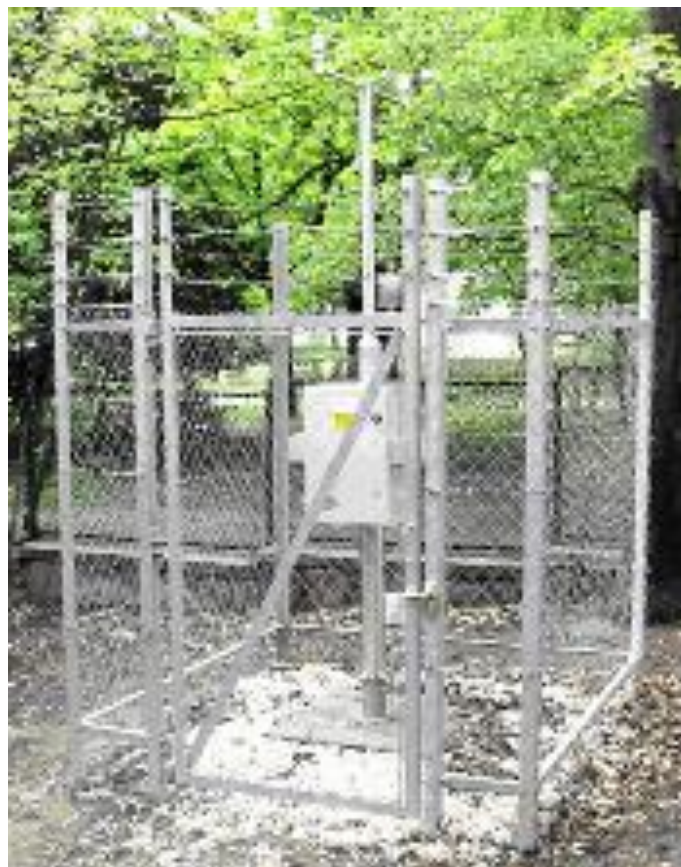
Figure 7. Deployed meteorological station with weather sensors
